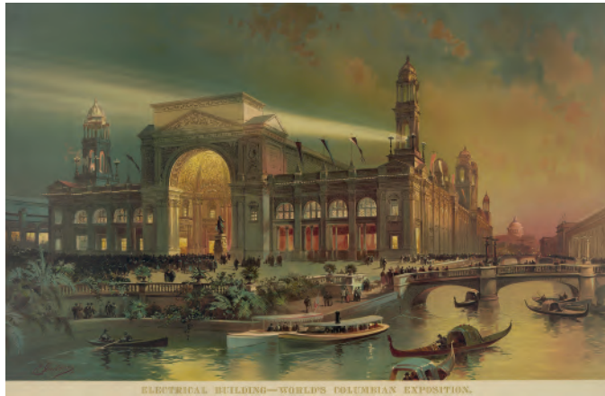
Electrical building, Chicago 1893 Everett Collection/Shutterstock.com
